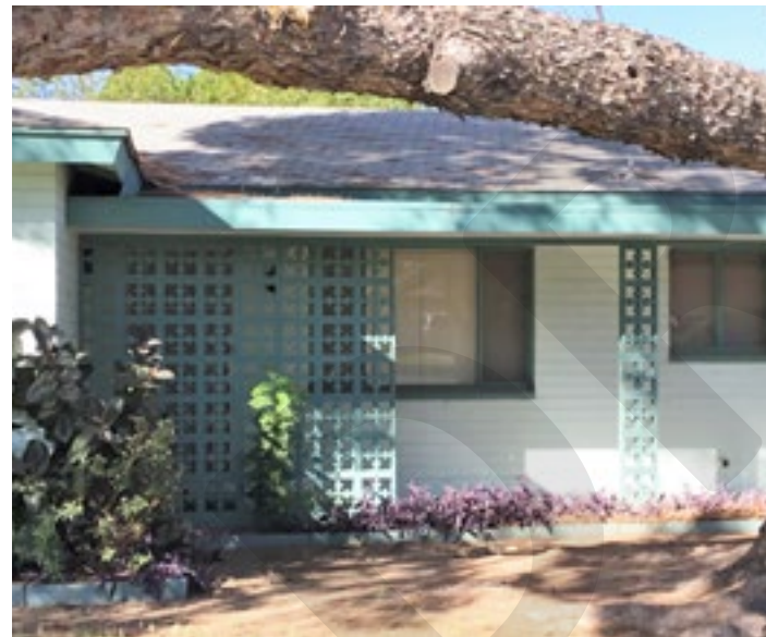
234 N. Fraser Dr. (The breezeblock elements on this porch contribute to the character of the house)
