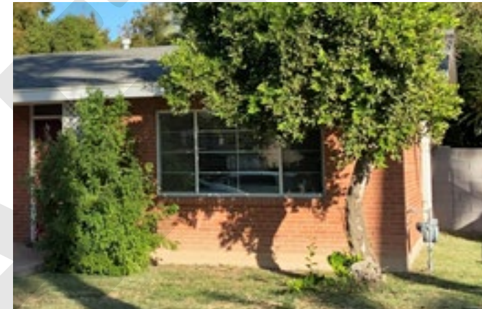
541 N. Grand (The foundation wall shown here uses different materials to visually distinguish it from the main wall)
