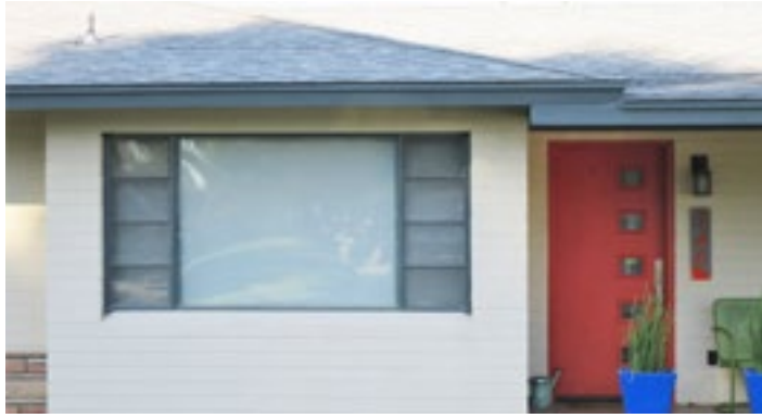
146 N. Fraser Dr. West (Original and historic doors help to convey the character of the style of the house)
