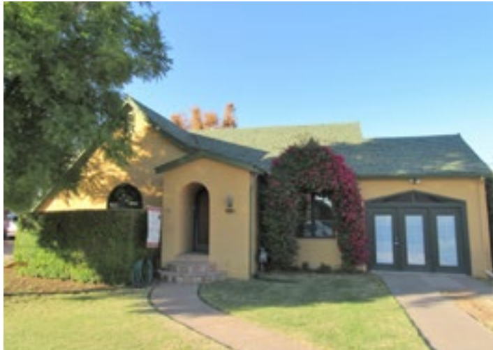
430 W. Clark (Garage enclosures, as shown here, should maintain the original door opening and use materials compatible to the house)
