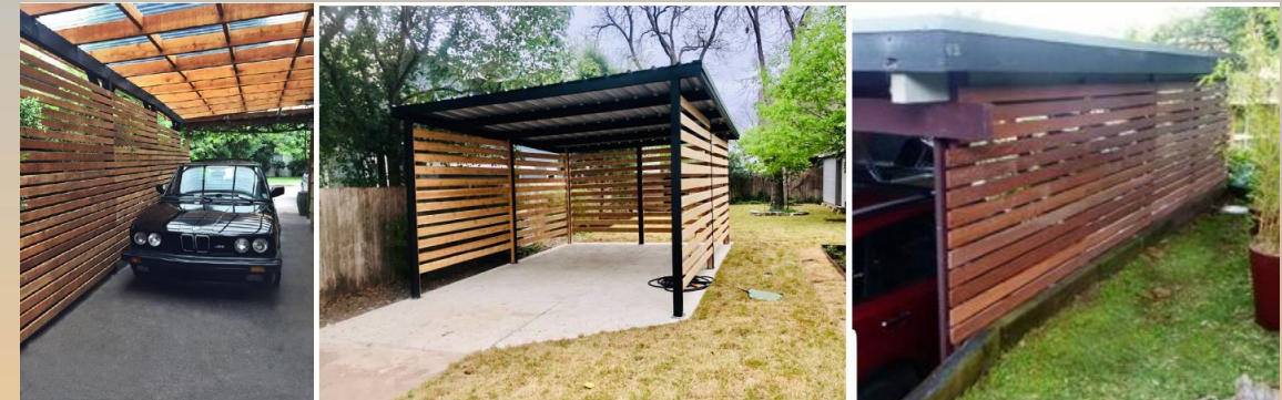
Images showing 6"x6" posts (used for guest house and carports) and wood slat walls (for carports)
