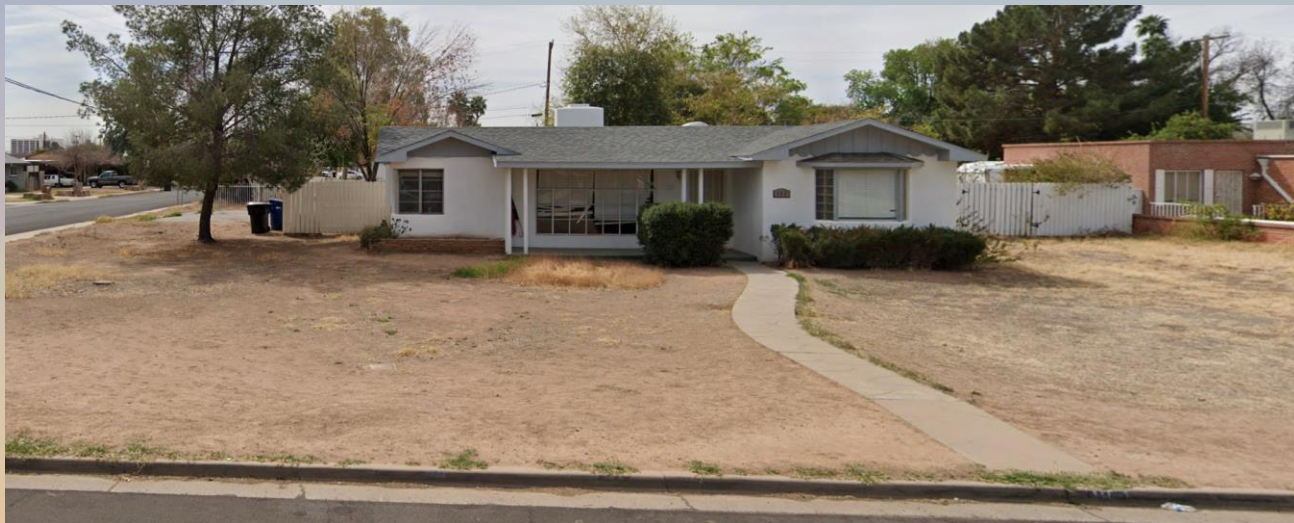
Front façade ca. Mar 2018
