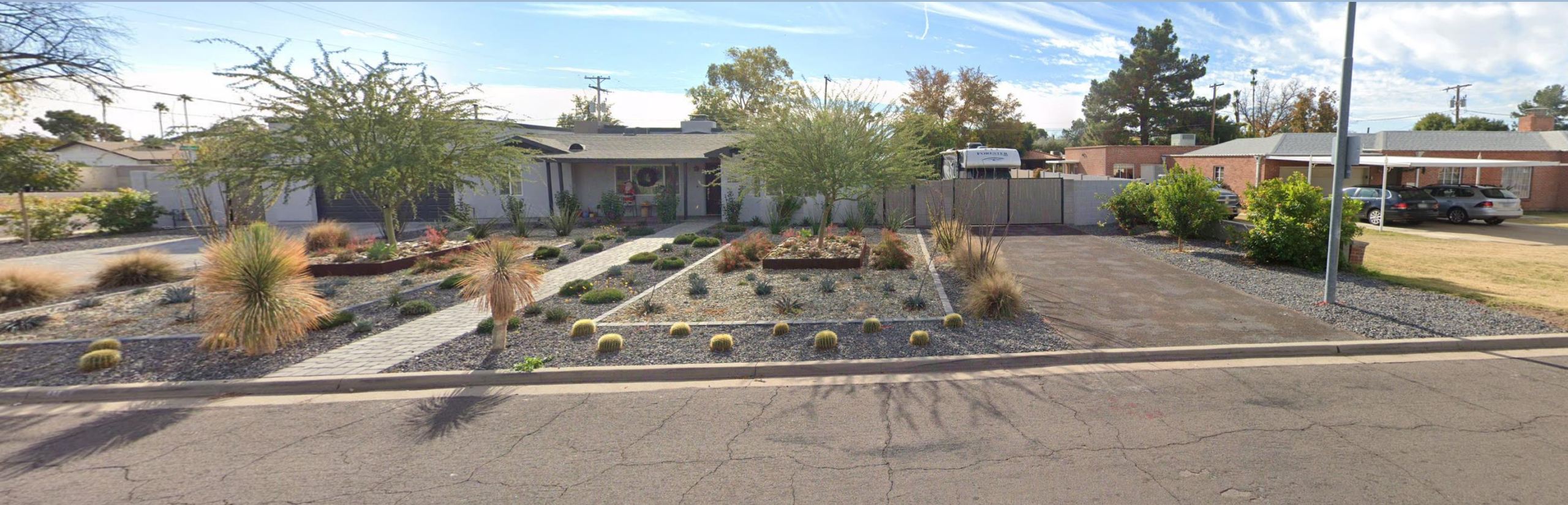
Front façade (north façade, looking south from W. 7 th Place)
