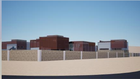
VIEW FROM CORNER OF MOUNTAIN ROAD AND PECOS ROAD LOOKING NORTHWEST - WITHOUT LANDSCAPING
