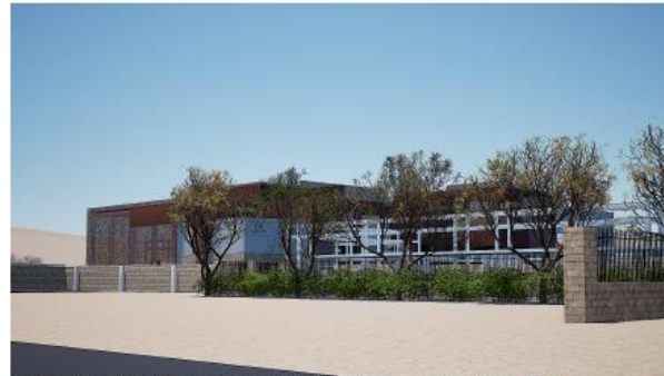
VIEW FROM MOUNTAIN ROAD LOOKING SOUTHWEST TOWARDS LOWER BUILDINGS - WITH LANDSCAPING
