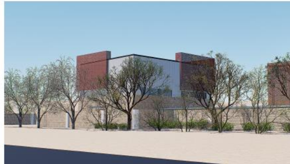
VIEW FROM MOUNTAIN ROAD LOOKING SOUTHWEST TOWARDS B-32 - WITH LANDSCAPING
