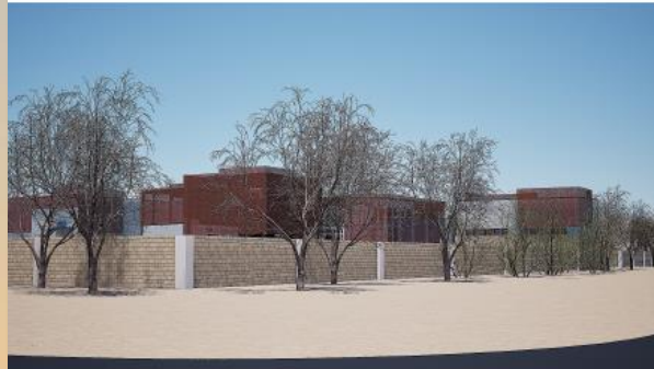
VIEW FROM CORNER OF MOUNTAIN ROAD AND PECOS ROAD LOOKING NORTHWEST - WITH LANDSCAPING
