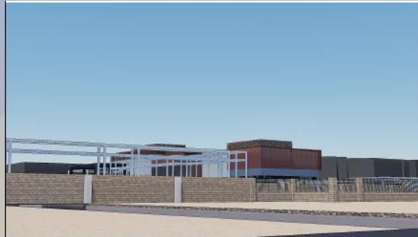
VIEW FROM MOUNTAIN ROAD LOOKING NORTHWEST TOWARDS UPPER GROUP OF BUILDINGS - WITHOUT LANDSCAPING
