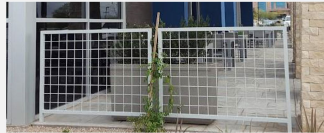
PATIO RAILING & WIRE MESH
