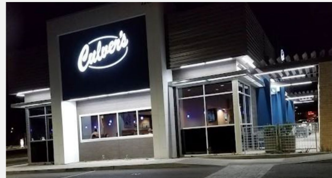
EXTERIOR LIGHTING LINEAR LIGHT FIXTURES
