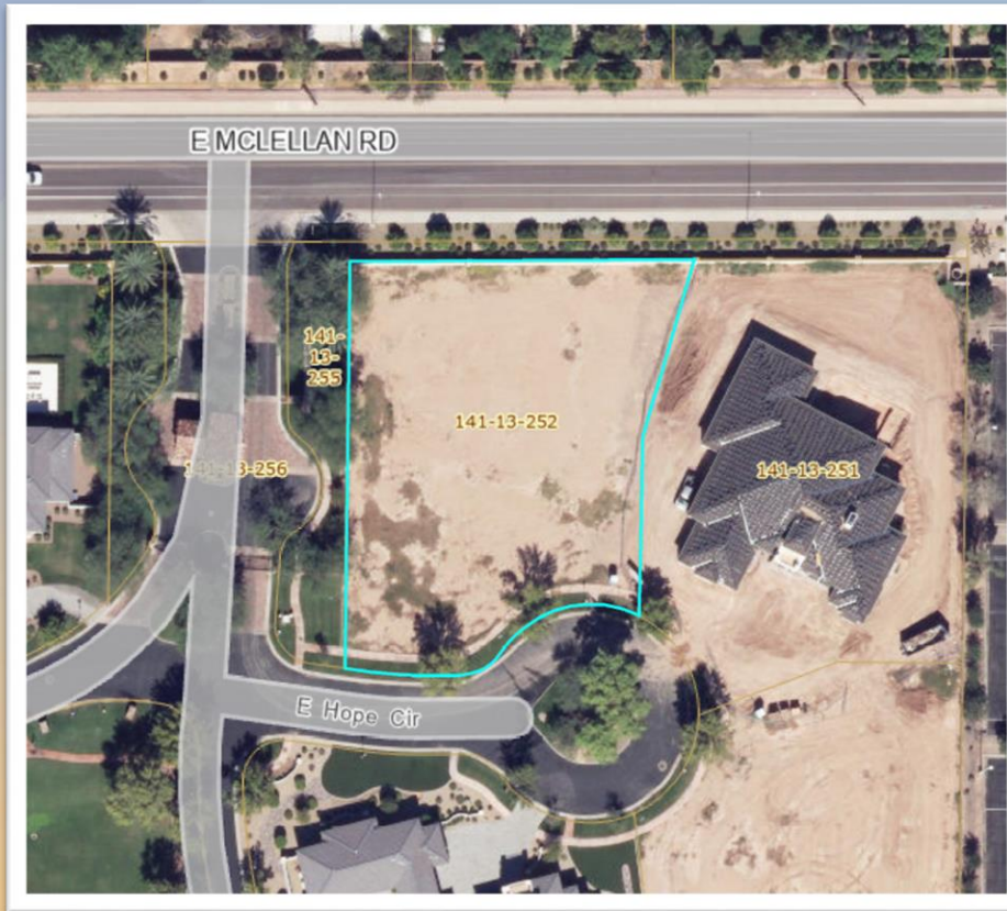
Aerial view of Lot 44 pre-construction
