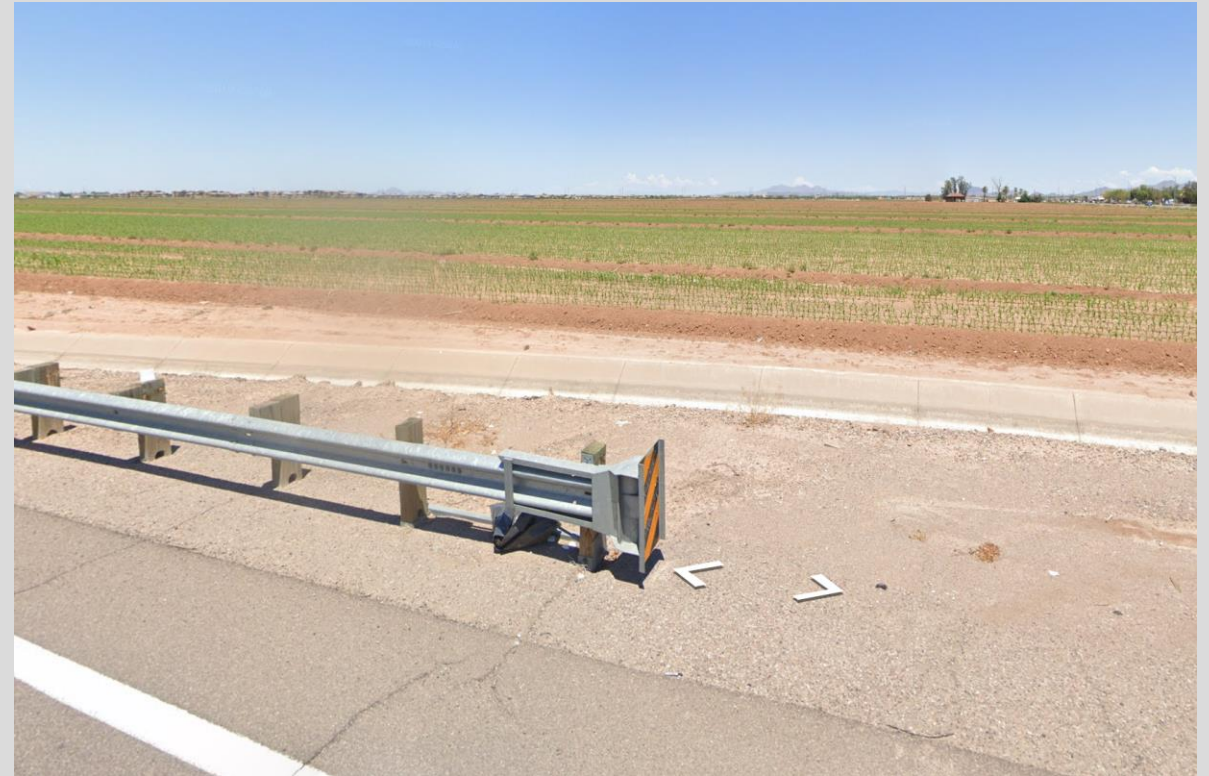
Looking south towards the site
