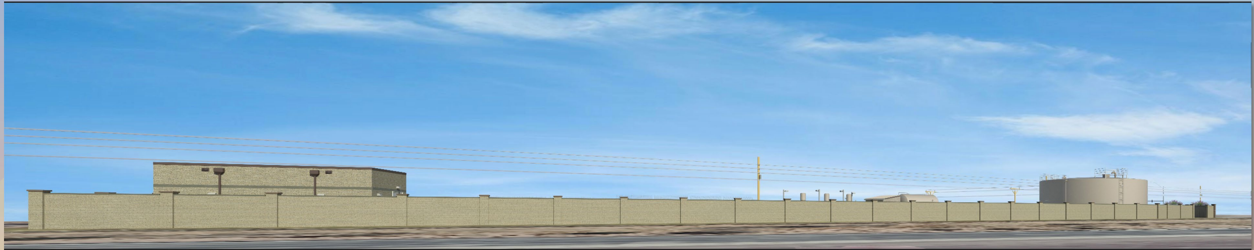
Looking south from the Loop 202
