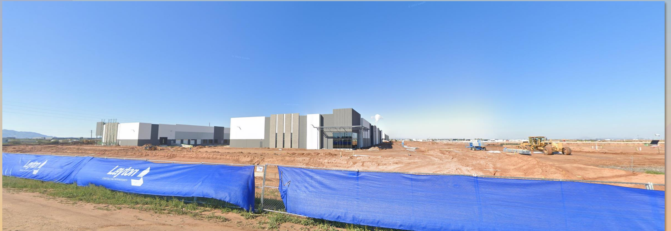
Looking southwest from S Sossaman Road
