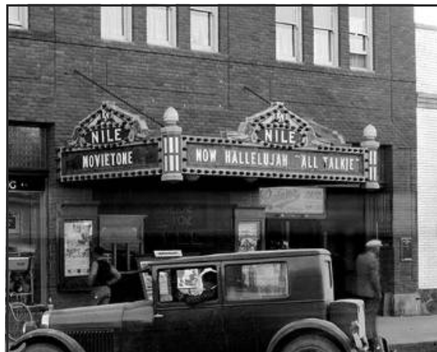
ORIGINAL MARQUEE SIGN
