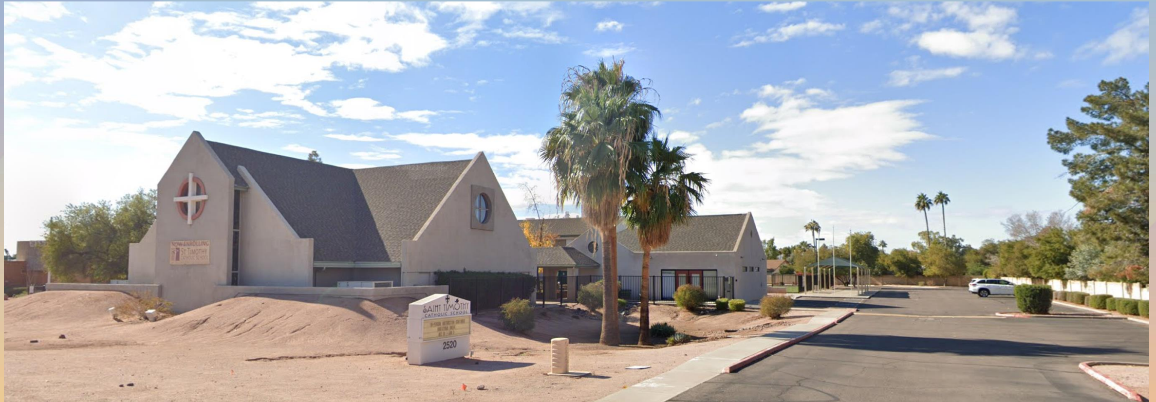
Looking southwest from Alma School Road
