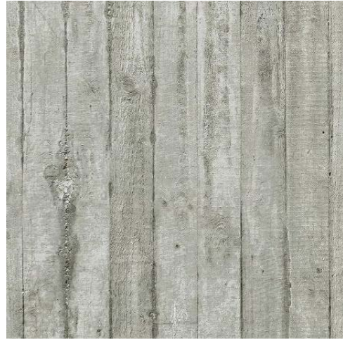
BOARD FORM CONCRETE
