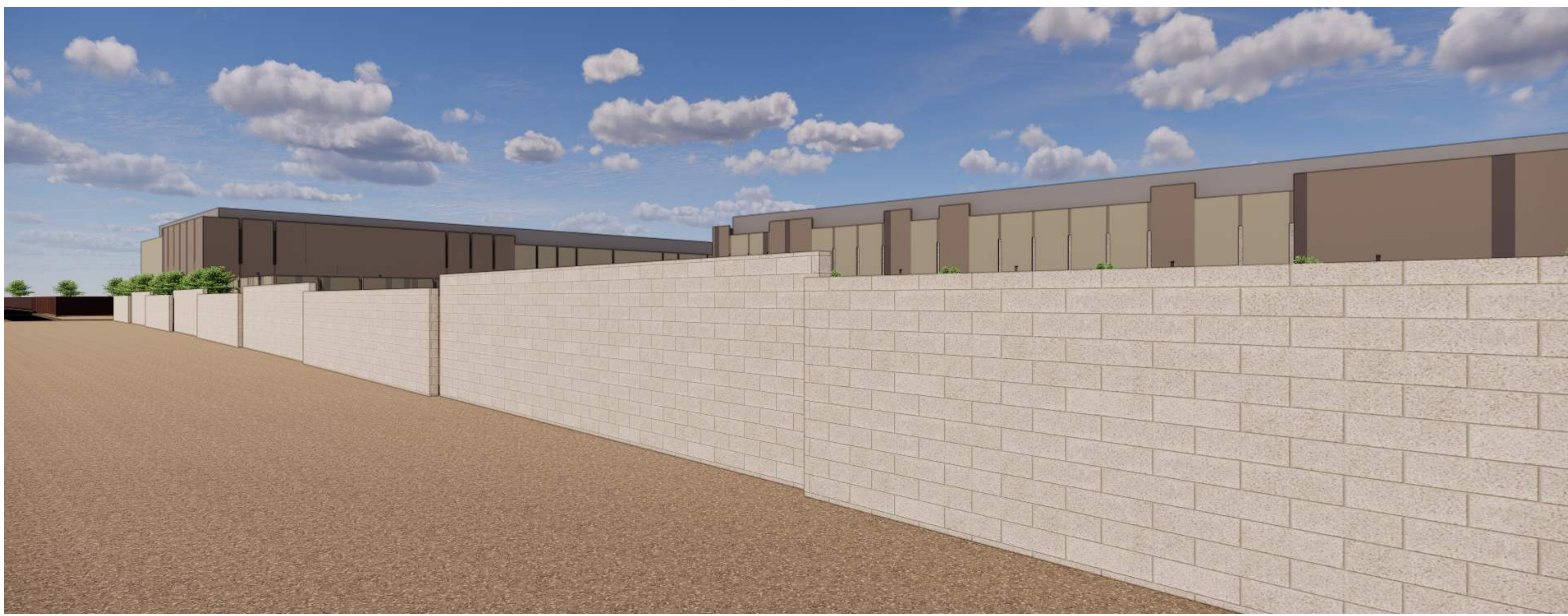
02 8' HIGH MASONRY ENCLOSURE WALL AT PROPOSED SUBSTATION
