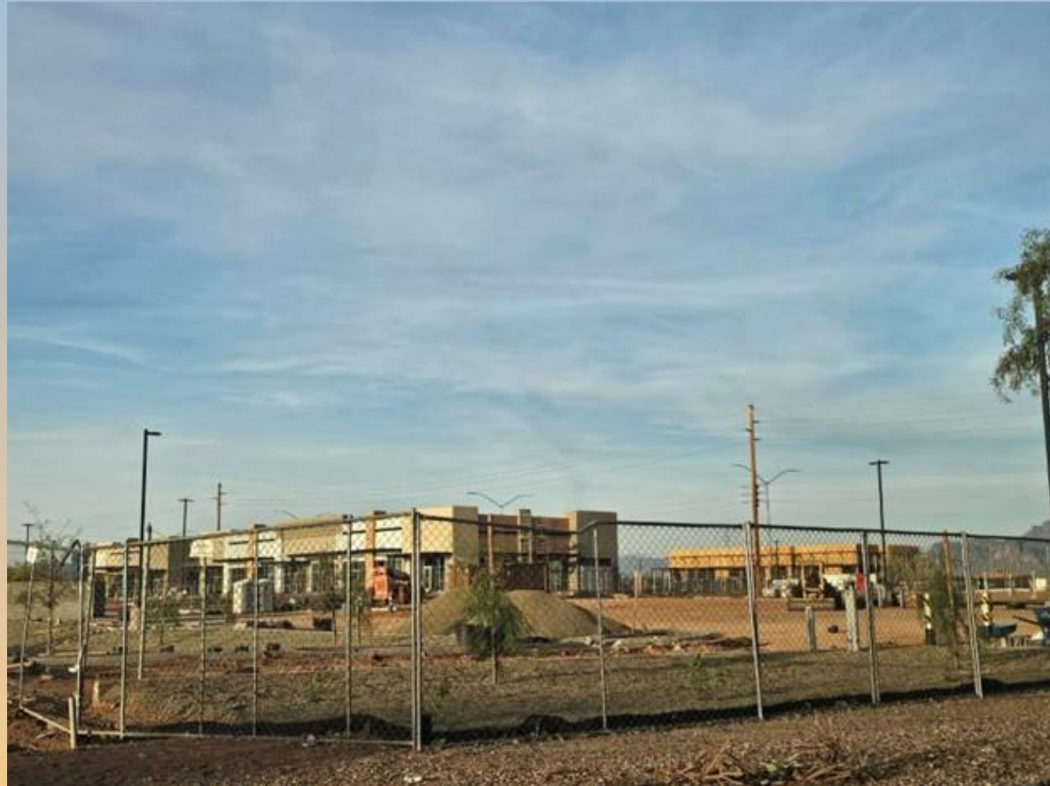
Looking northeast from the hospital parking lot
