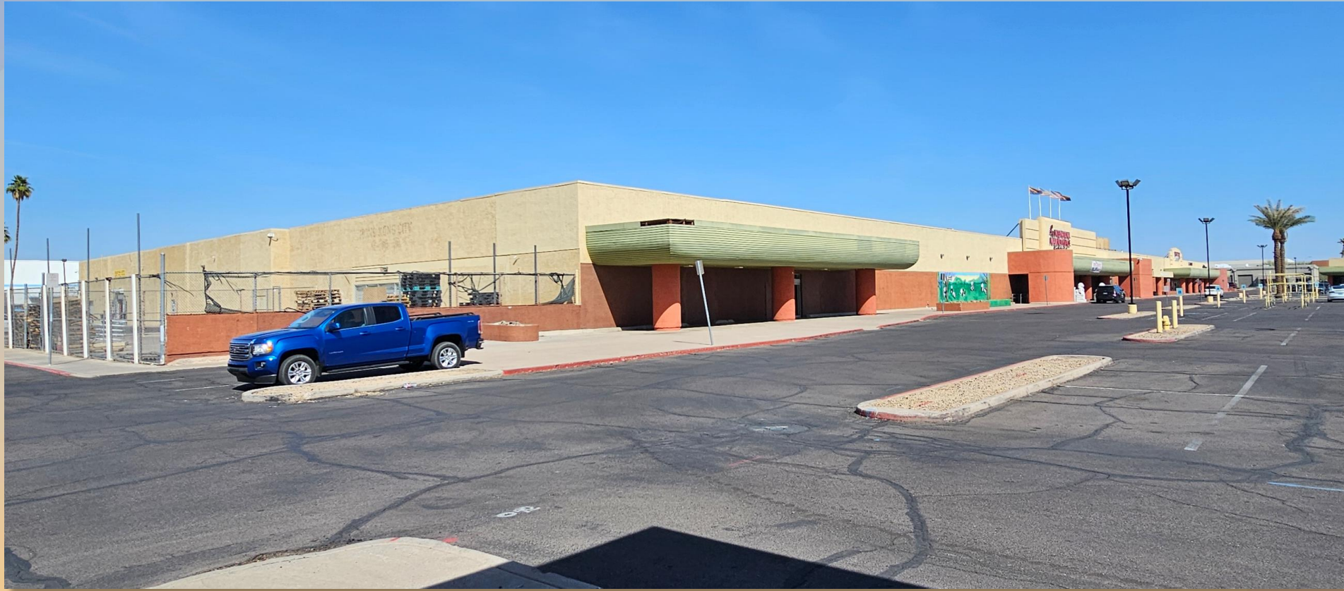
West end of building, looking northeast from Dobson Rd
