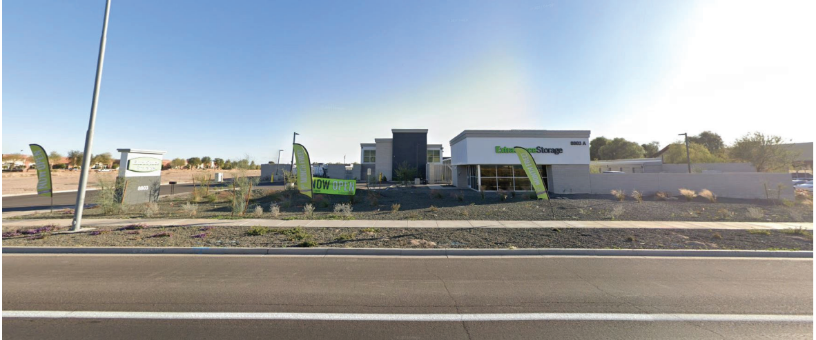
Image 1: Extra Space Storage, Williams Gateway Self Storage (APN# 304-62-942). Existing self-storage property located directly west of the proposed development, utilizing similar materials of concrete masonry, metal paneling, and stucco, as well as similar color palette.
