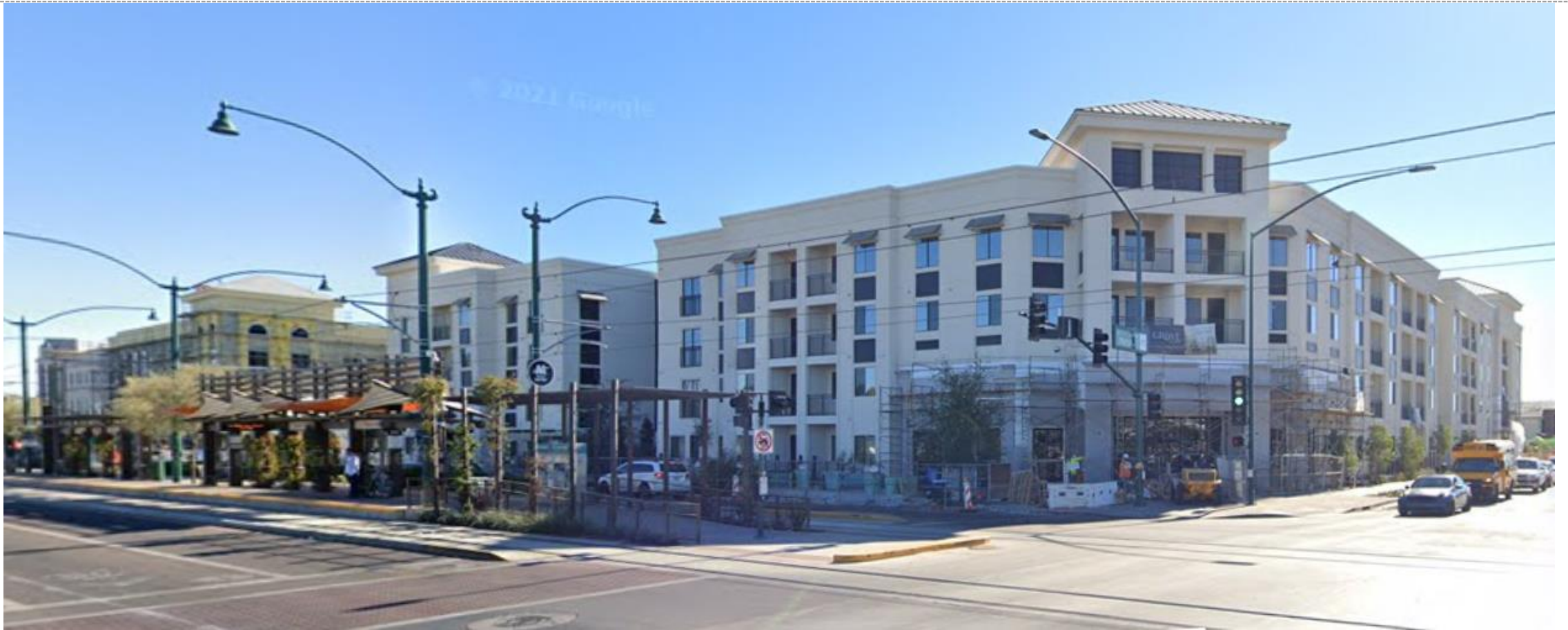
Looking southeast from Mesa Drive and Main Street
