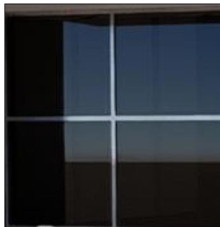
AL-01: KAWNEER NORTH AMERICA ALUMINUM STOREFRONT "CLEAR ANODIZED FINISH" TO MATCH ADJACENT SUPERMARKET
