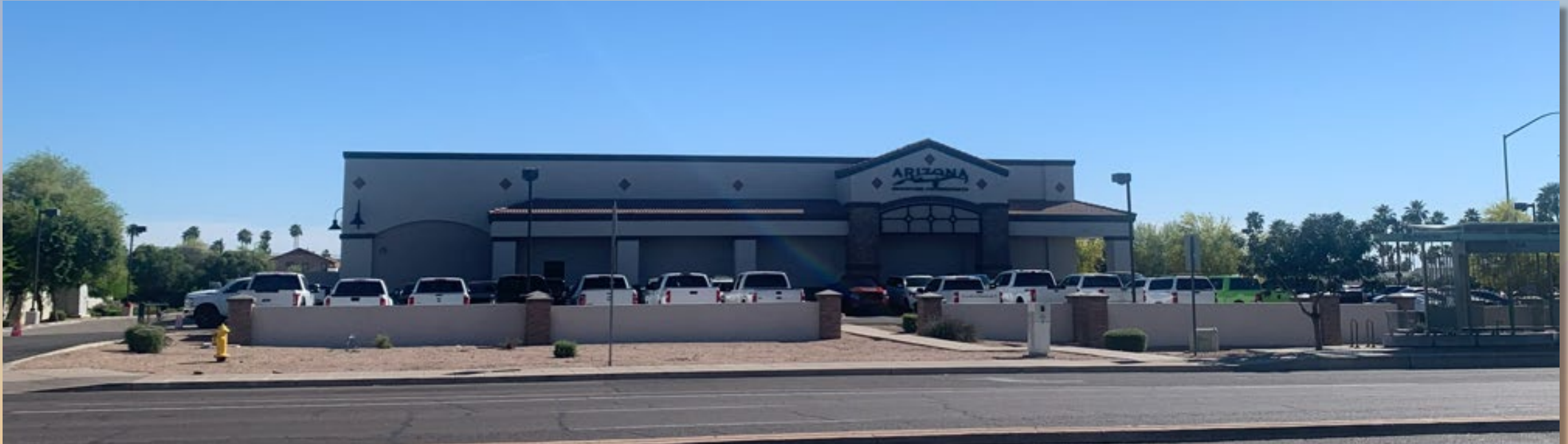
Looking South from Main Street
