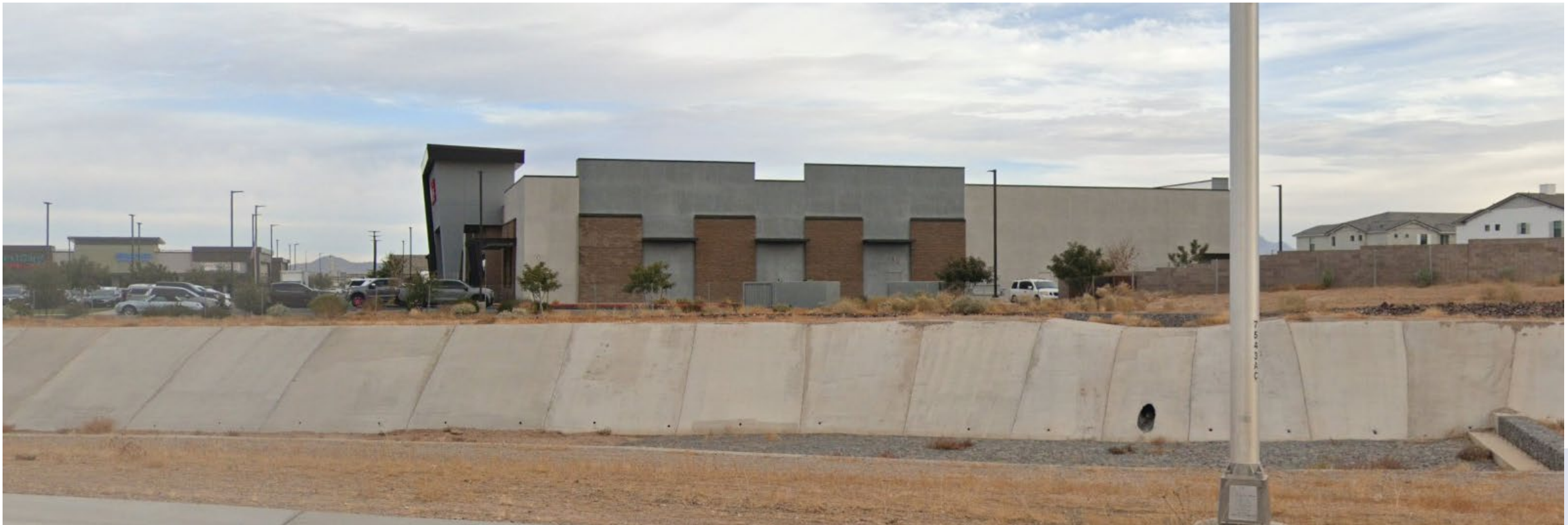
Looking north towards the site from the SR-24 Freeway
