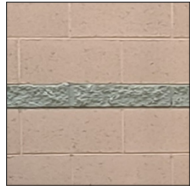
MATERIAL M2 BROWN-GRAY SPLIT FACED CMU 16X8 - ACCENT SINGLE ROW ECHELON (OLDCASTLE) "GRAY" COLOR
