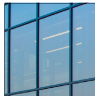
MATERIAL M6 BLACK ANODIZED FRAMES WITH VITRO SOLARGRAY 1" INSULATED GLAZING WINDOWS AND GLAZED DOORS EXTERIOR LIGHTS TO BE BLACK ANODIZED
