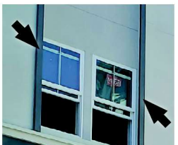
9. ARCHITECTURAL TRIMS TO MATCH PAINT SPEC E
