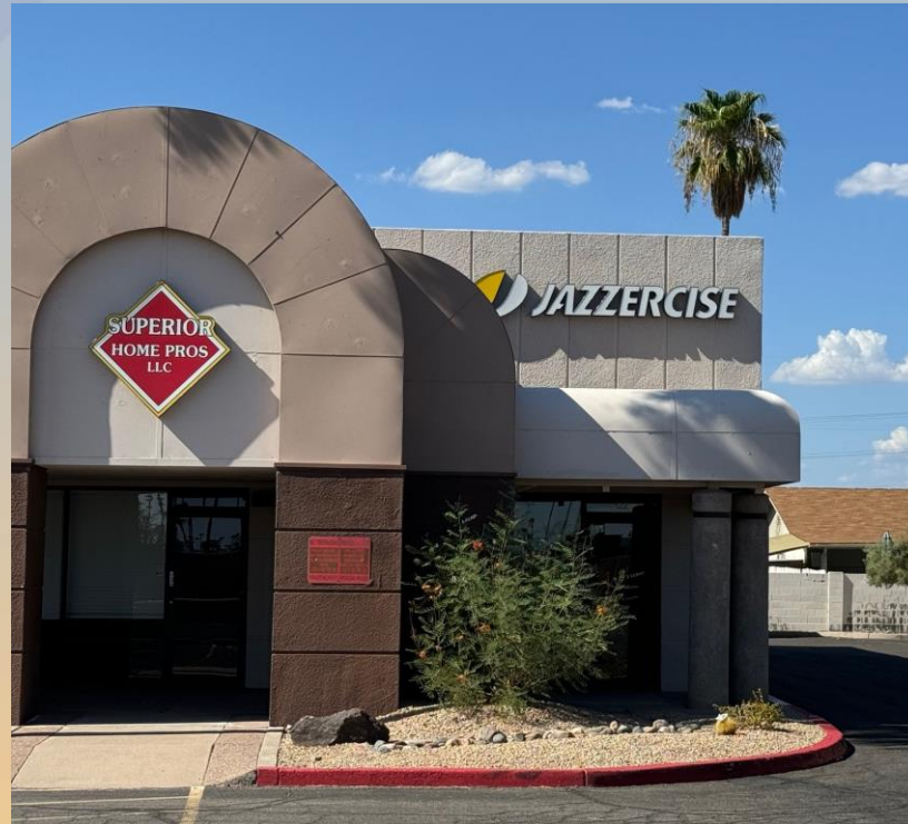
Front of Building
