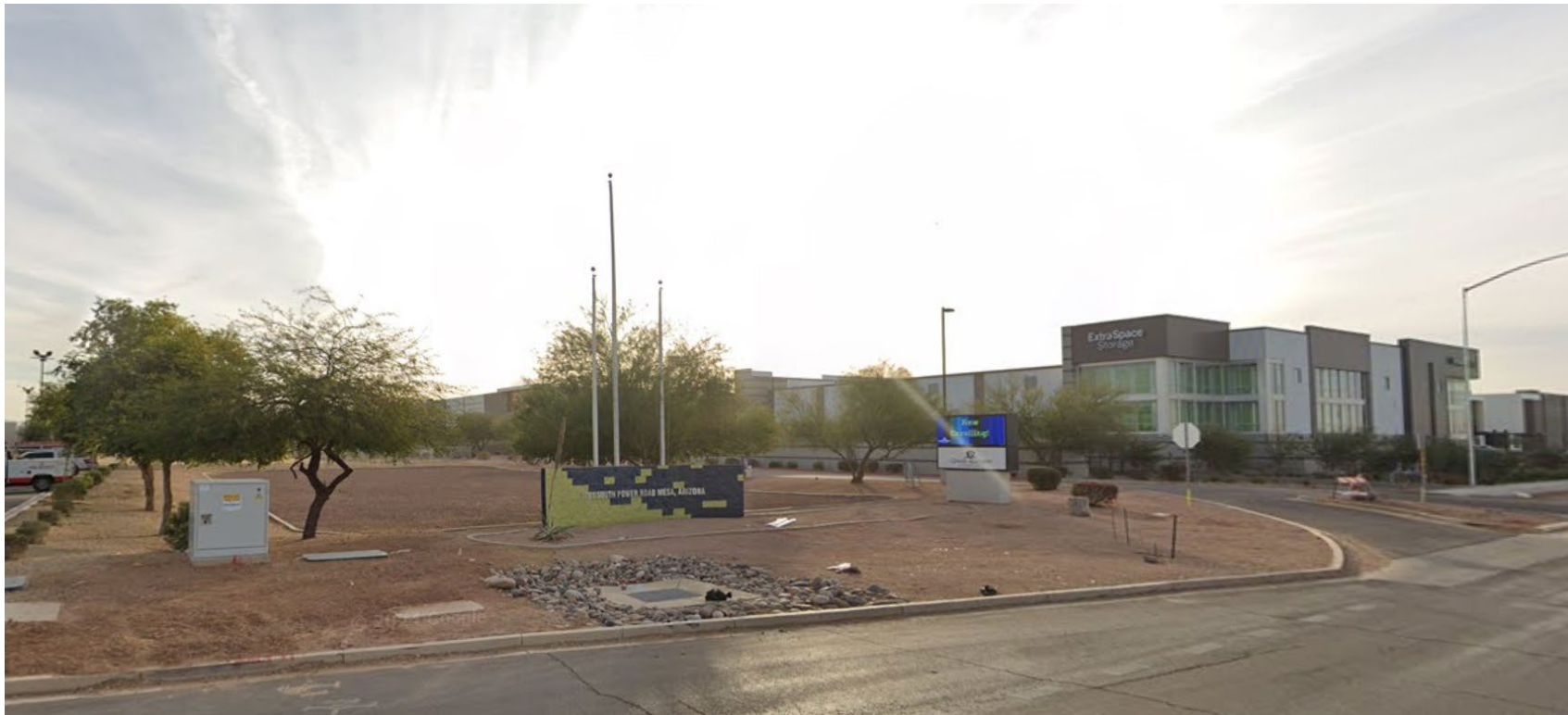
Looking East from Power Road
