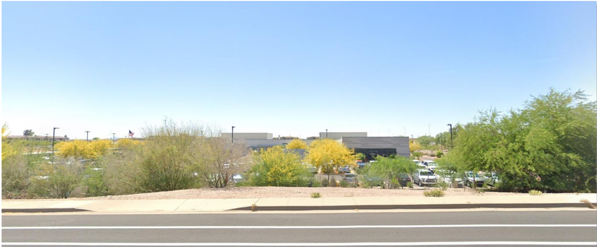
Looking west towards the site
