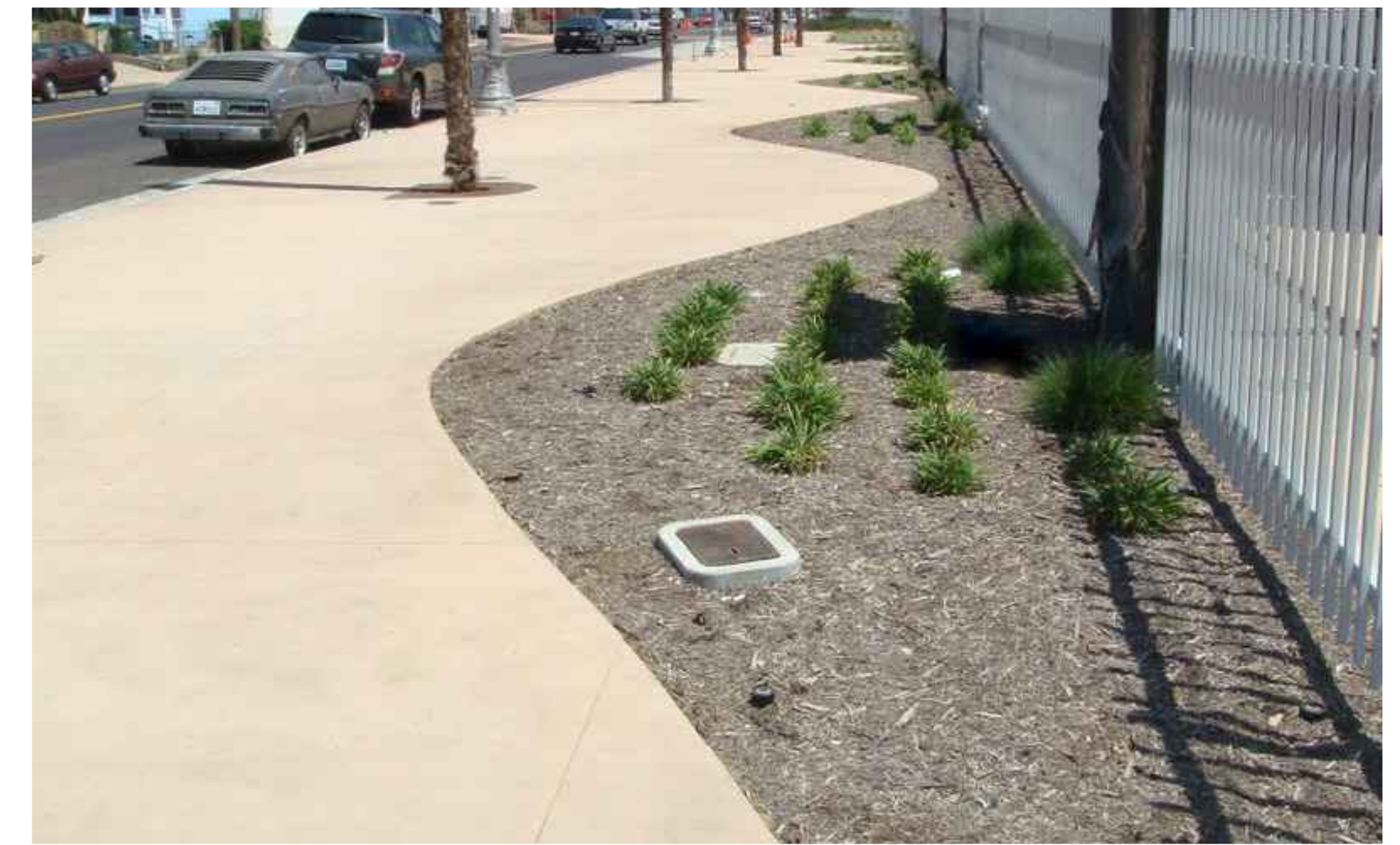
INTEGRAL COLORED CONCRETE
