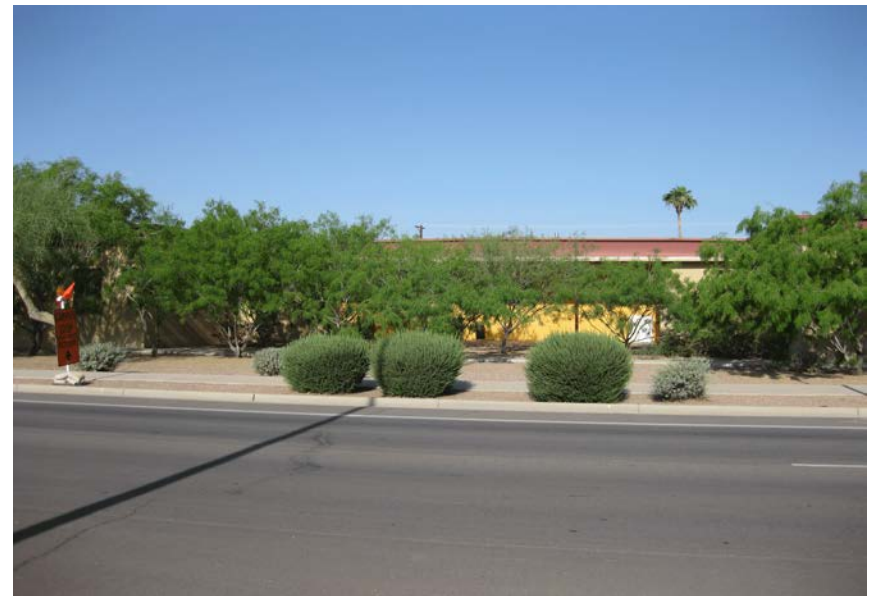
Ground View – East Side of Building
