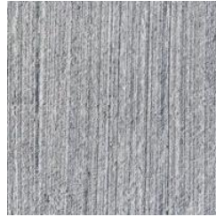
BROOM FINISH CONCRETE
