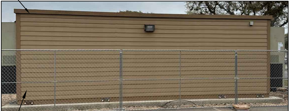
NORTH ELEVATION PHOTO
