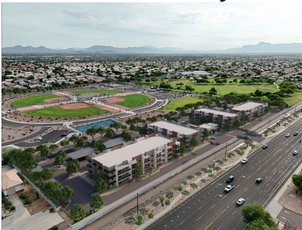
NEC Power & Guadalupe Roads (Mesa, Arizona)
