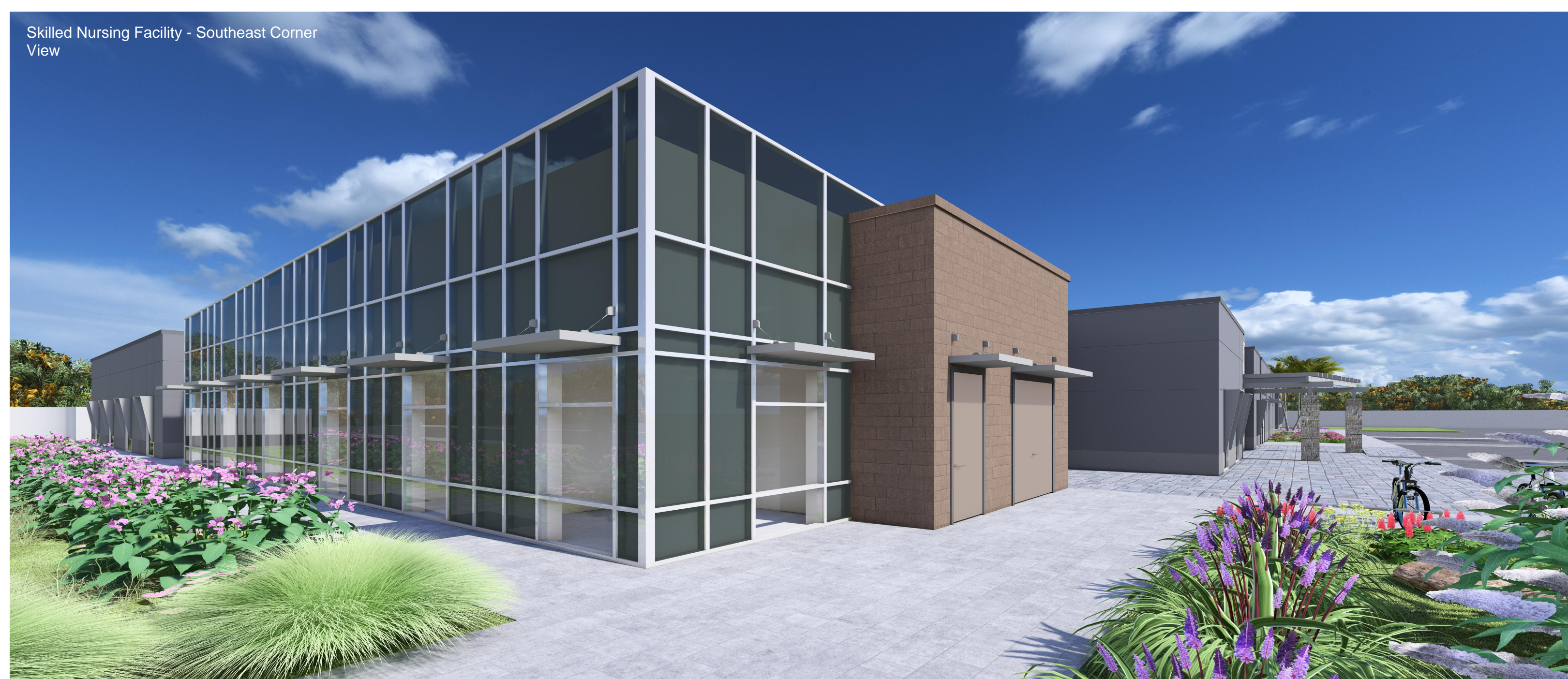
Skilled Nursing Facility - Front Looking at the Entrance
