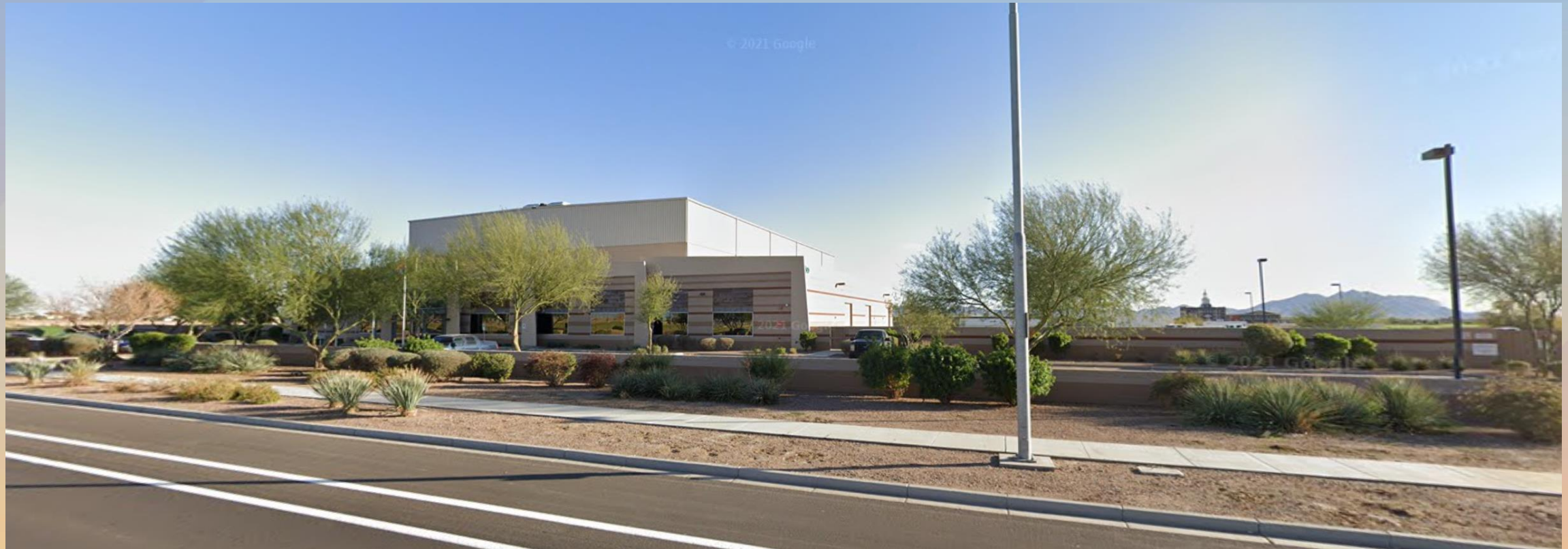
Looking southeast at the existing Metso site
