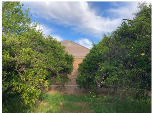
Existing House (looking East)
