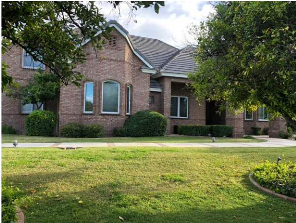
Existing House (looking Southwest)
