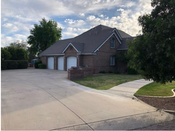
Existing House (looking Southwest)
