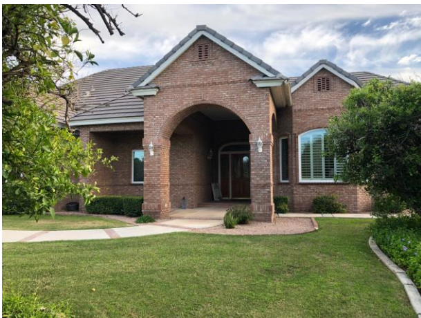
Existing House Entrance (looking South)
