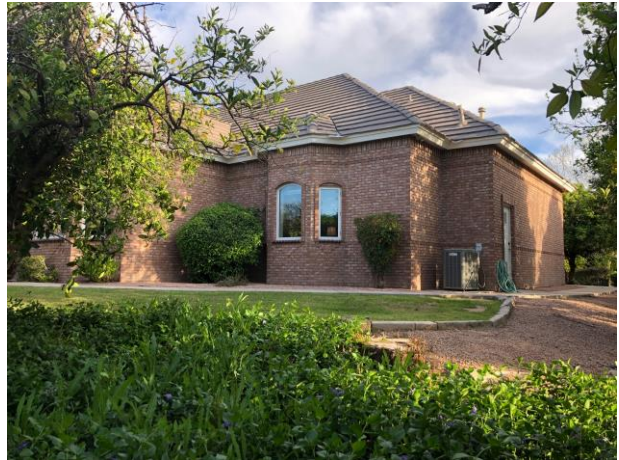
Existing House (looking Southeast)
