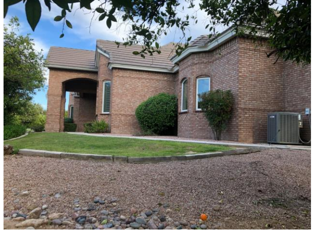
Existing House Entrance (looking East)
