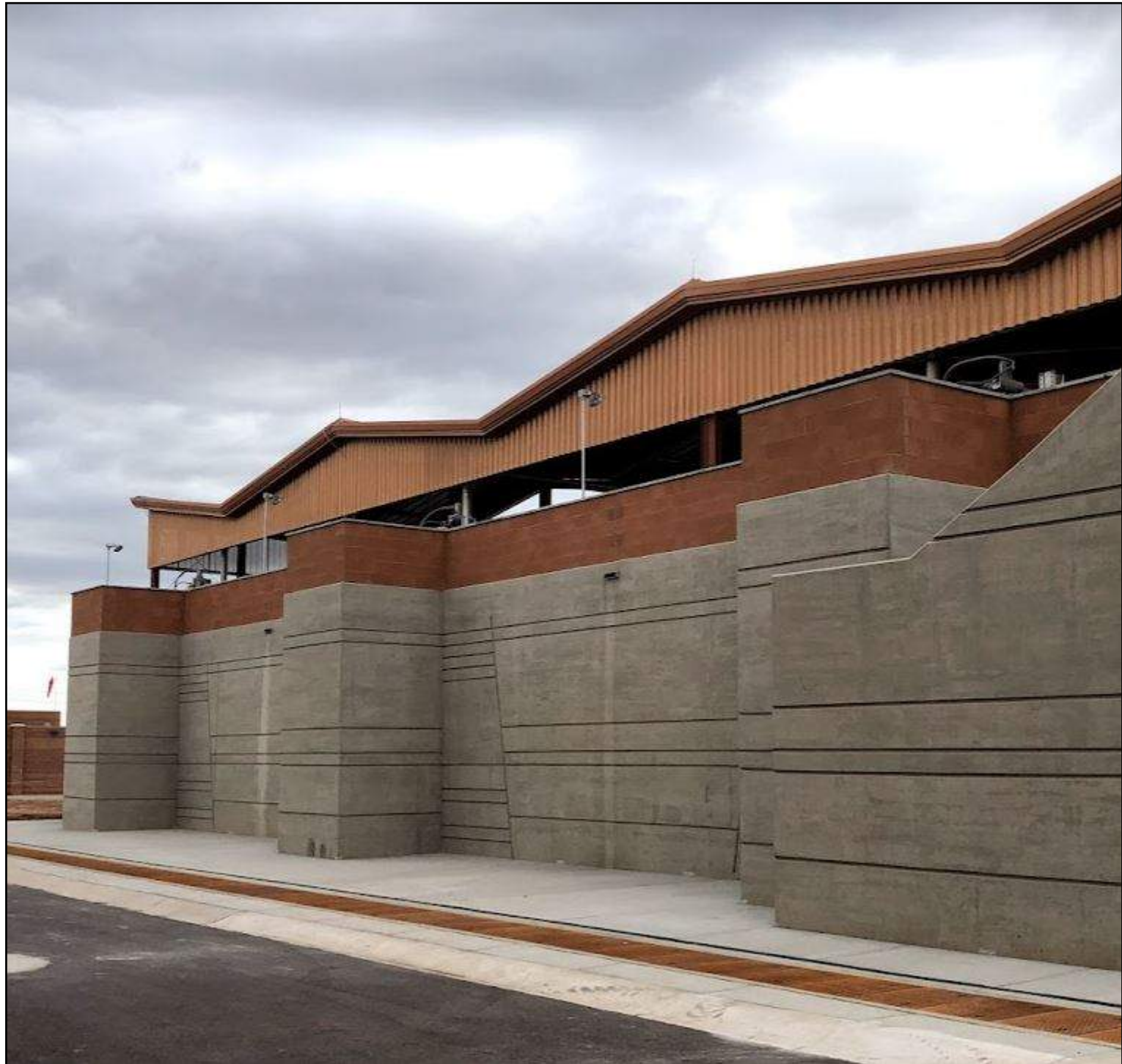
Existing Filter Complex
