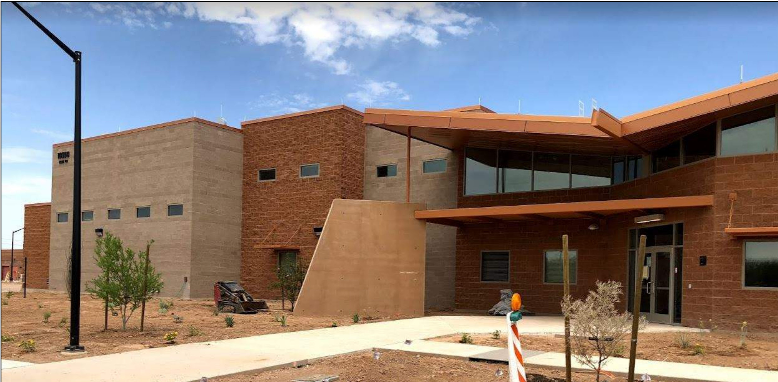
Existing Operations Building
