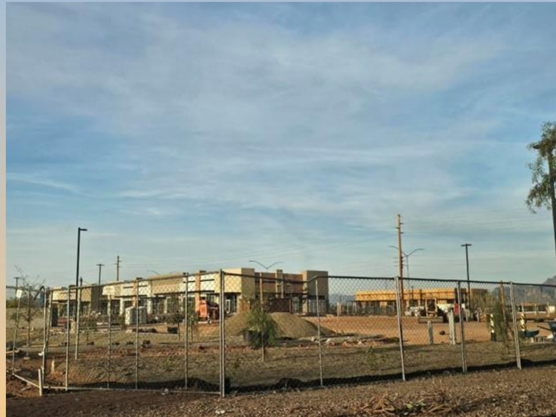
Looking northeast from the hospital parking lot
