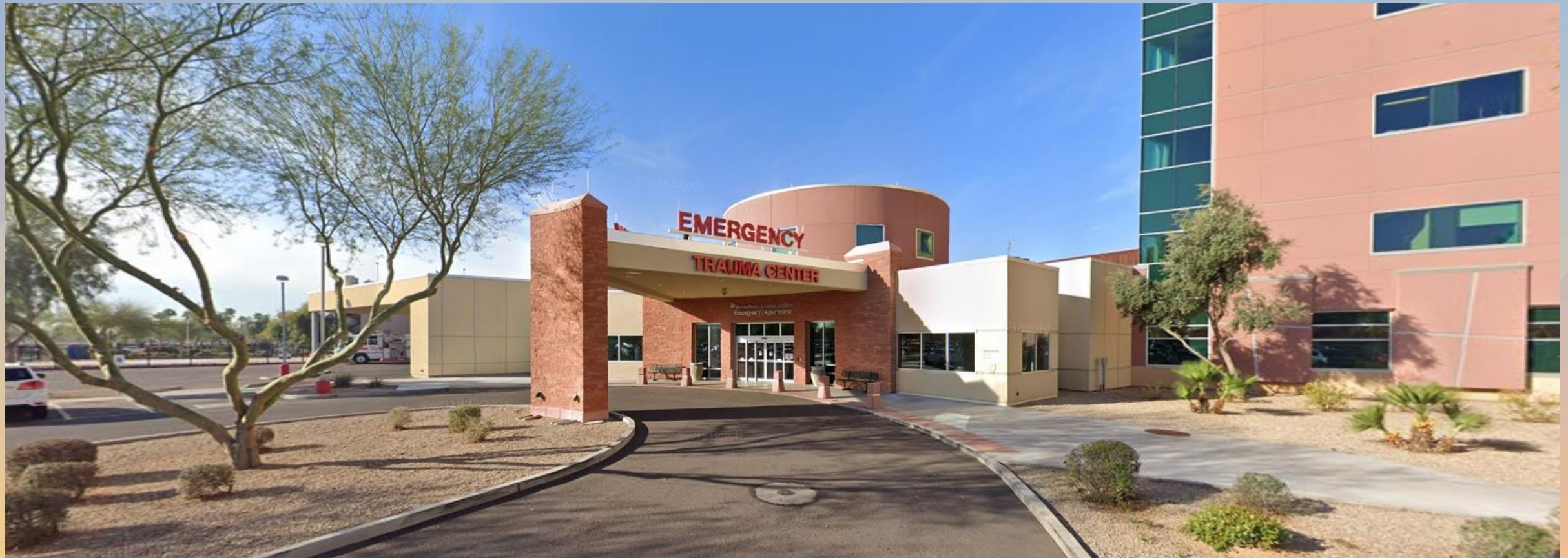
Looking west towards the site from an internal drive aisle
