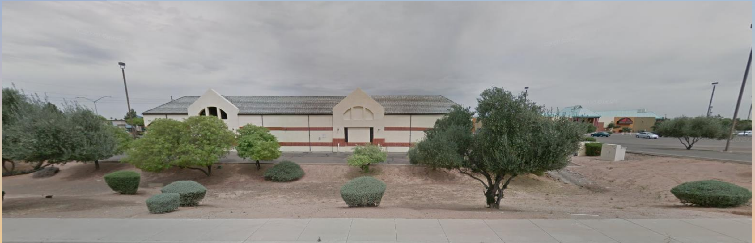
Looking north from Kiowa Avenue
