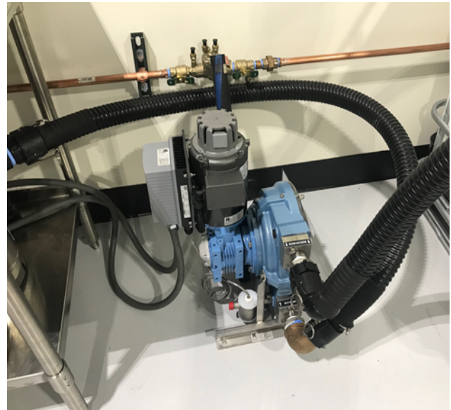
Figure 4: Peristaltic pump
