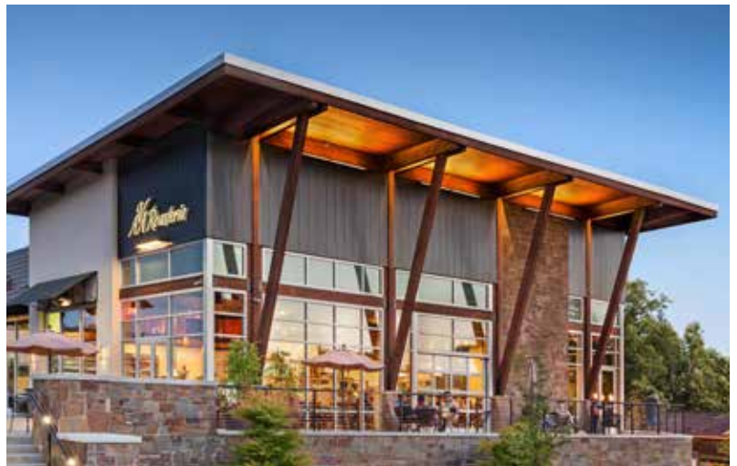
clarity of contemporary materials with protected wood soffits
