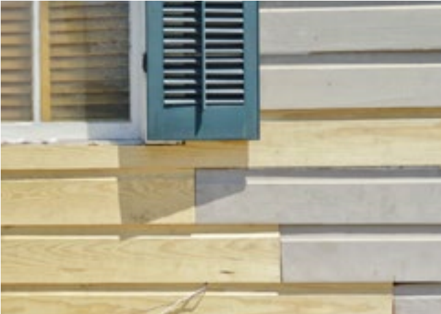
The Dutchman repair method allows for the installation of new wood while preserving the historic wood.
