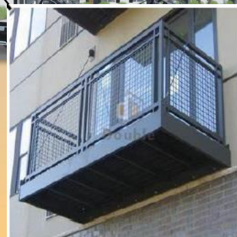
WIRE MESH RAILING
