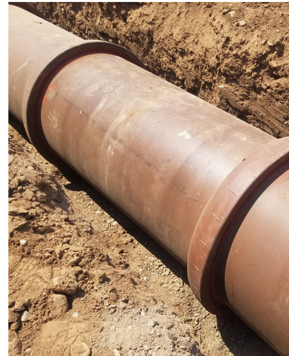
New Sewer Mains
