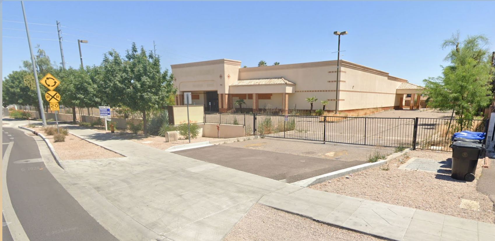
Looking south from Main Street
