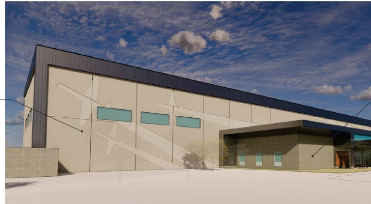
Southwest perspective, flight graphics integrated into tilt-up wall panels (final graphics TBD)
