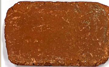
BRICK VENEER USED OVER FRONT FACADE CMU WALL
