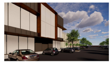
05 BUILDING ENTRY OVERHEAD
