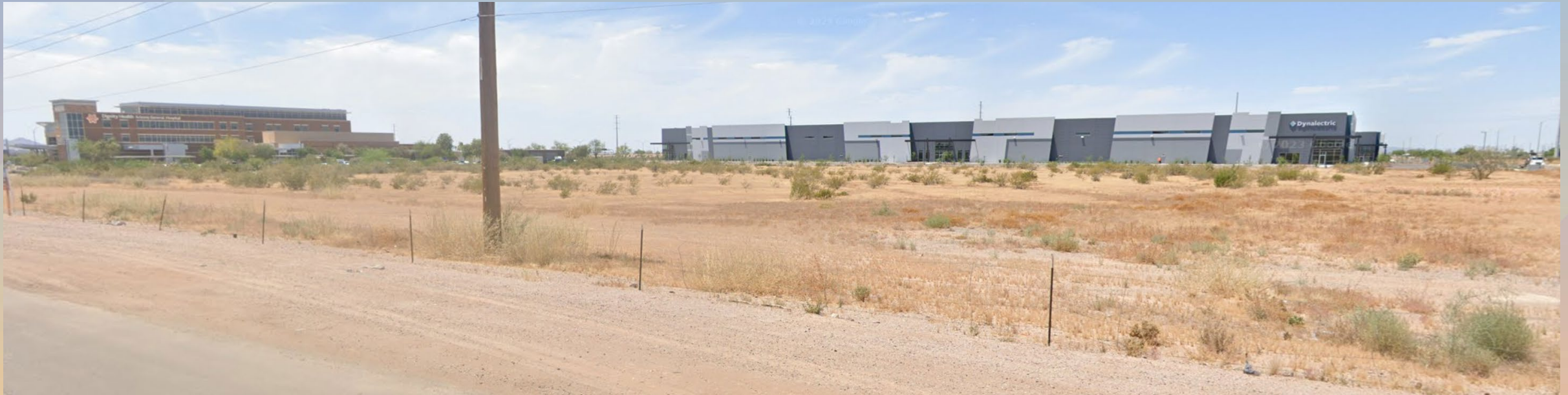
Looking southwest from Ellsworth Road
