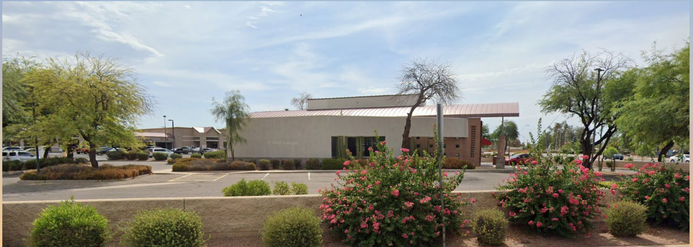
Looking east towards the site from Power Road
