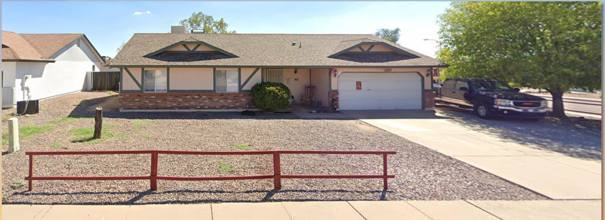
Looking south from Halifax Street
