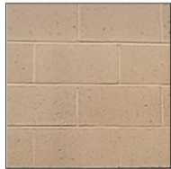
MATERIAL M1 BROWN STANDARD FINISH CMU - 16X8 RUNNING BOND ECHELON (OLDCASTLE) "PEBBLE" COLOR
