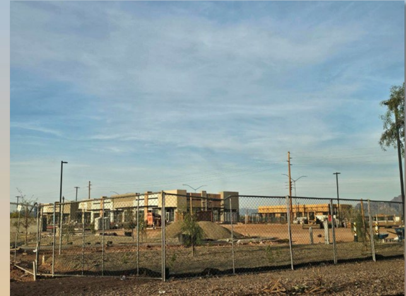
Looking northeast from the hospital parking lot
